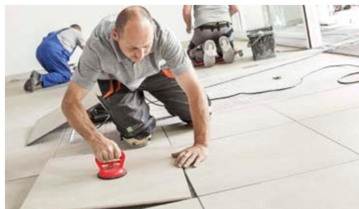
5 DryTile tiles can be easily replaced at any time. Simply cut open the joint, remove the tile with a suction lifter and insert the new tile.
