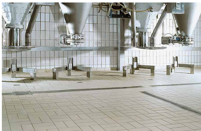
Production hall, Nuremberg, Germany
