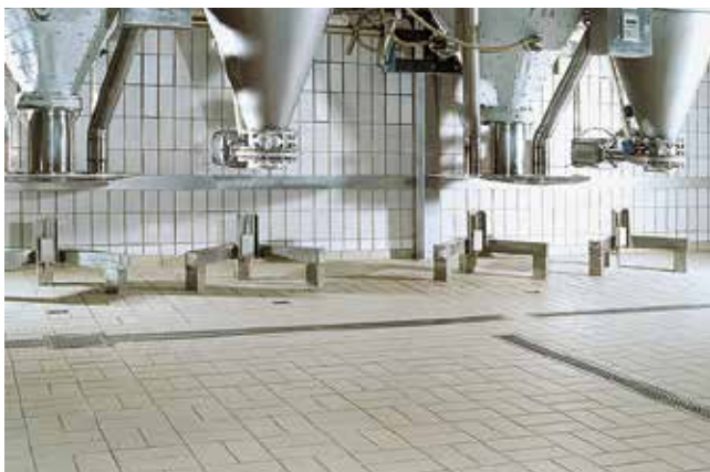
Production hall, Nuremberg, Germany
