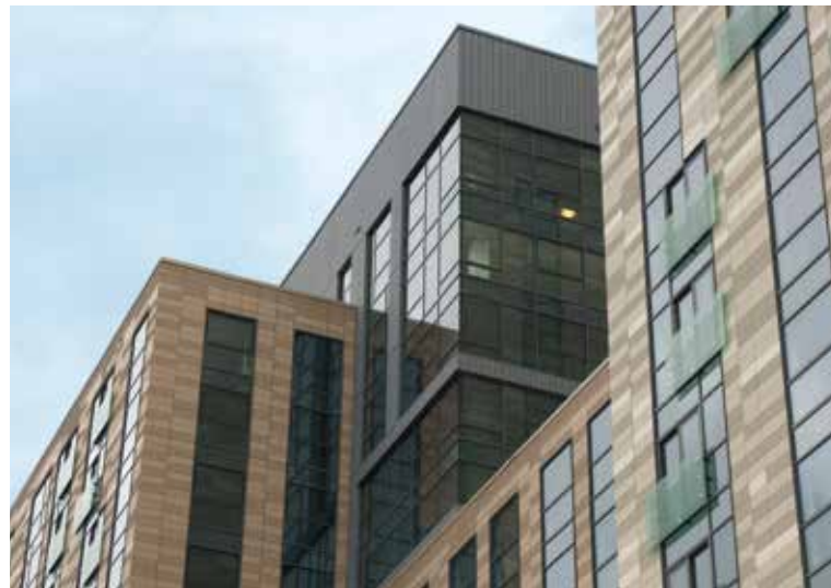
The Viridian, Boston, EE UU / Arquitecto: Bruner/Cott & Associates / Foto: Fred Clements / LEED GOLD
