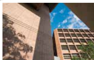
Lee Shan Building, Hong Kong, Cina
