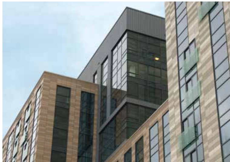
The Viridian, Boston, USA / Architetto: Bruner/Cott & Associates Foto: Fred Clements / LEED GOLD
