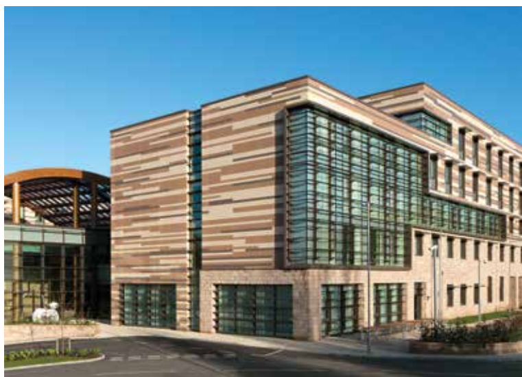
Orchard Hotel, Nottingham, Gran Bretagna / Architetto: RHWL Architects Foto: Martine Hamilton Knight Photography / BREEAM EXCELLENT
